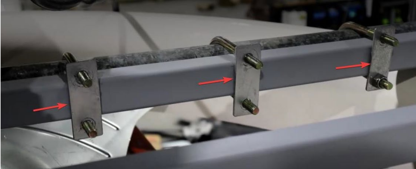
10. Thread and tighten the nuts on each end of the U-clamp.
